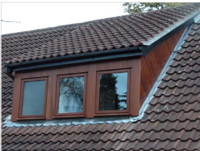
Catslide dormer extension
